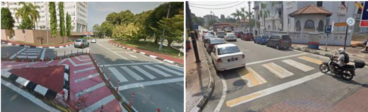
Fig. 1: Example of Pedestrian walkways with curbs that end abruptly without curb cuts at zebra crossings. No tactile paving was installed for the blind. Confusing Zebra Crossing. (Source: Author)
